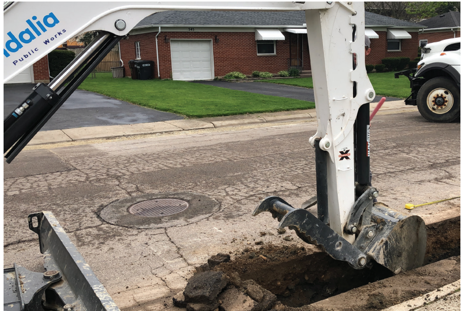
Repairing a watermain break is a big job. First, crews need to excavate the road to expose the break below.
