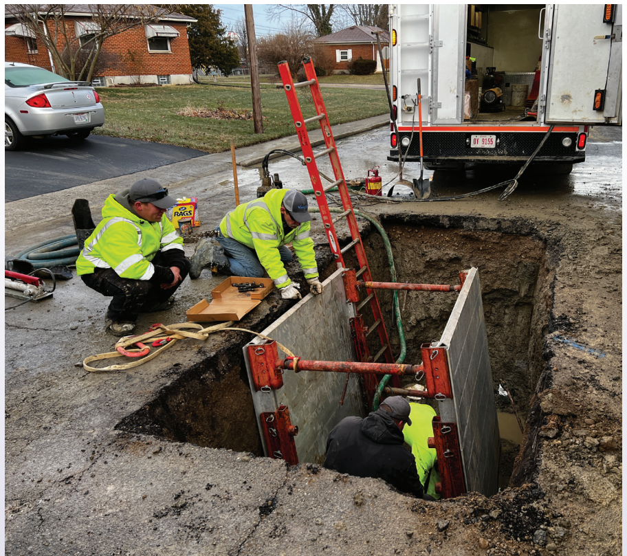
Once exposed, crews secure the work area and begin the task of repairing the break.
