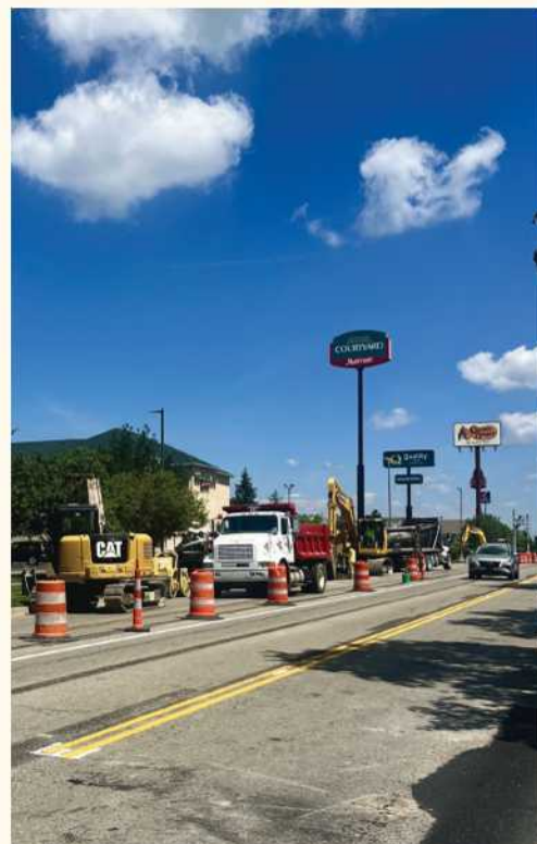
Crews have completed concrete work on the East side of Miller Lane and have now transitioned to the West side of Miller Lane to complete repairs.
