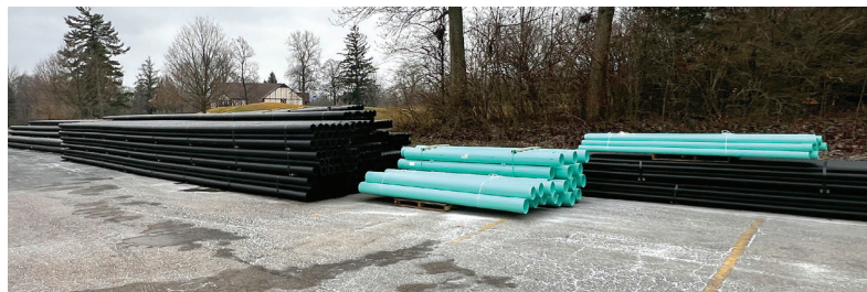
Irrigation lines have been staged at the golf course for installation this summer.
