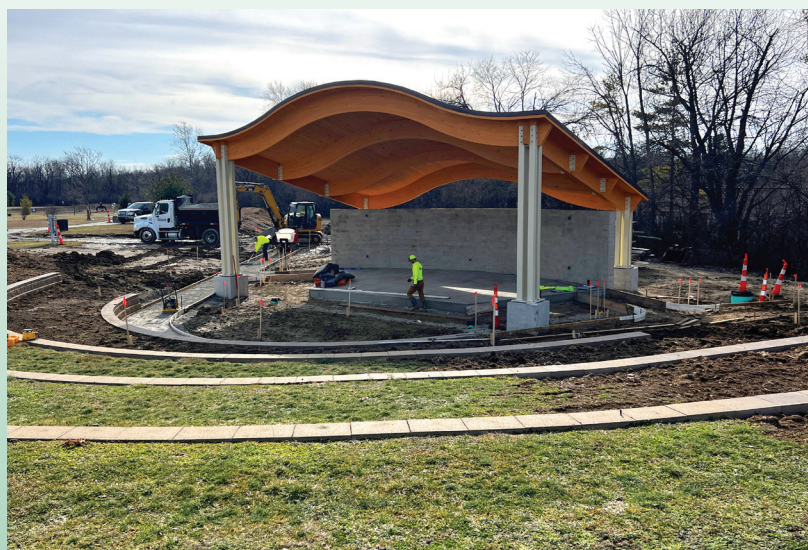
New amphitheater stage is under construction.
