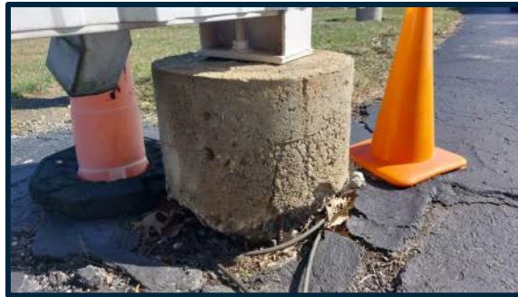
Damaged Concrete Piers
