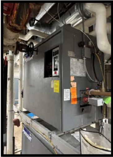
Existing Boiler prior to removal
