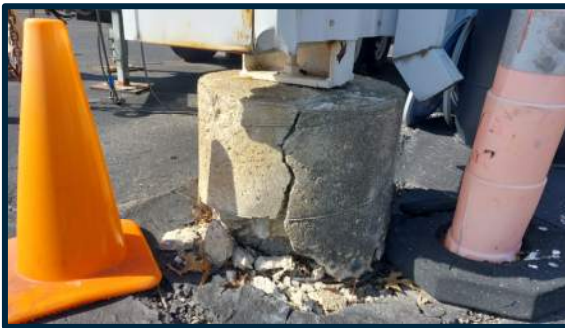
Damaged Concrete Piers
