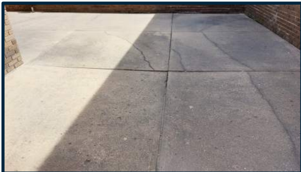
Basement Areaway Concrete
