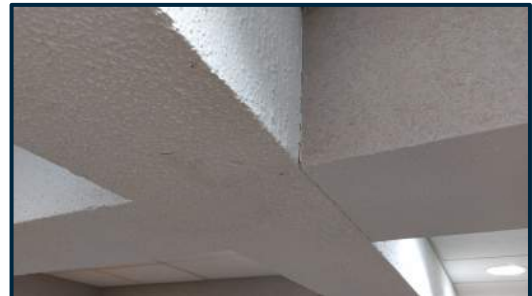
Textured Finish on Beams
