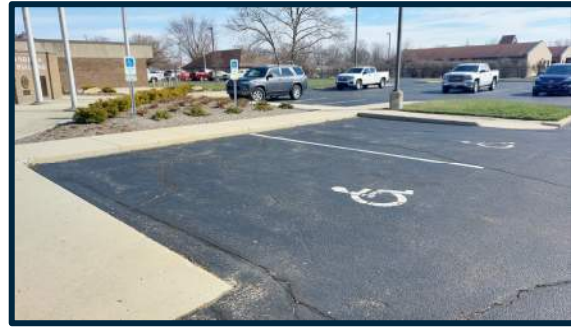
Existing Handicapped Parking Spaces
