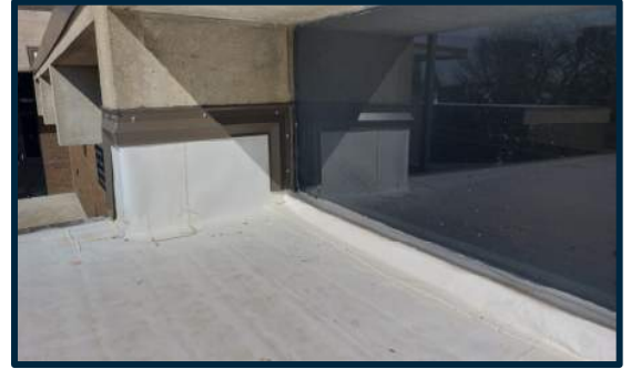
Short Roof Flashing at Clearstory Windows
