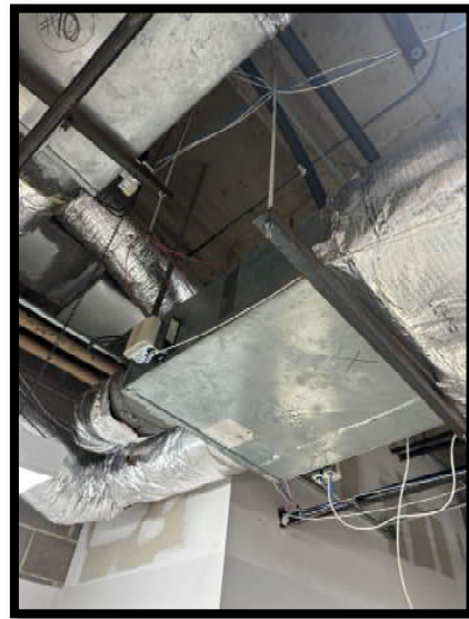
Typical Dual Duct VAV Terminal Unit
