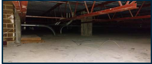
Recessed Floor Infill from Below
